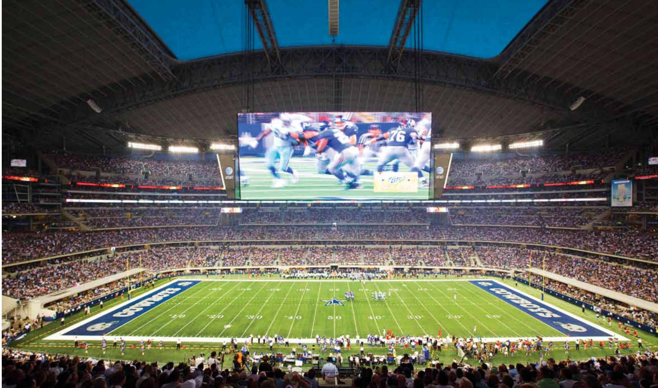
The stadium's retractable roof section is composed of twin mechanized translucent panels that slide lengthwise across the top of the dome. Suspended from the roof's arch trusses 90 ft above the field is the world's largest high-definition video screen system.
