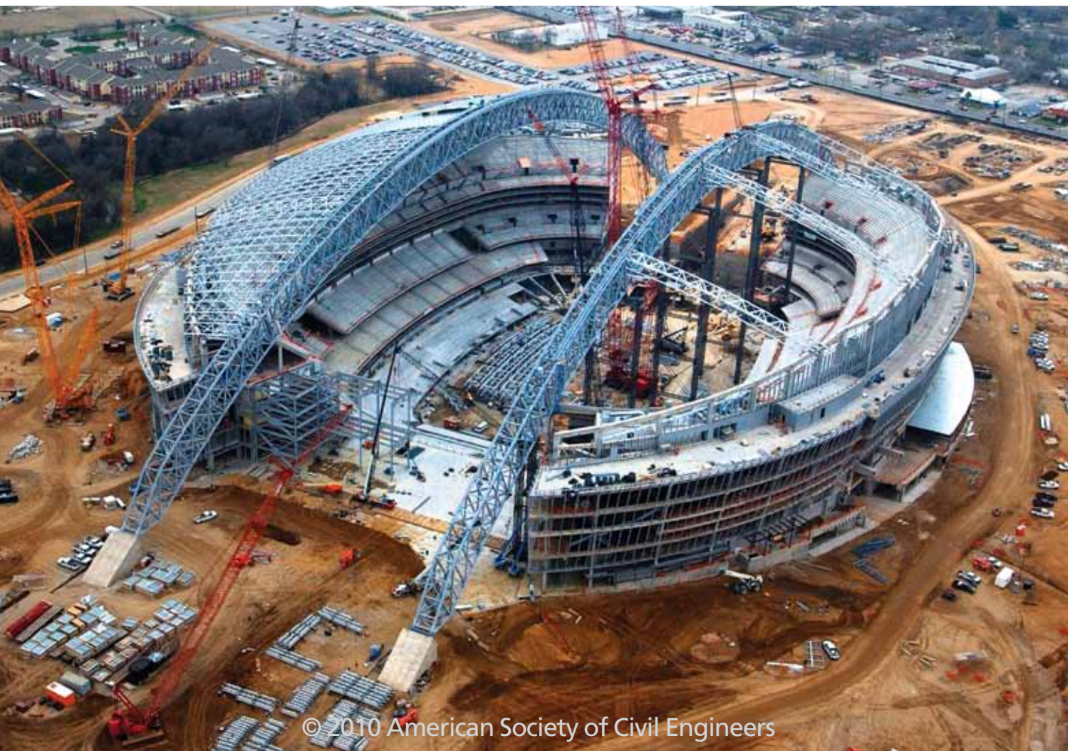
COURTESY MANHATTAN CONSTRUCTION COMPANY/PHOTO BY AERIAL PHOTOGRAPHY, INC.
